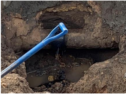
a. Buried pipes and cables
