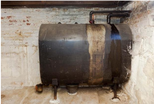
a. Old tanks being removed
