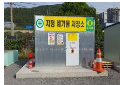
Hazardous waste storage area
