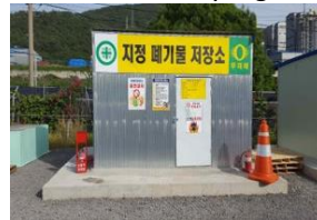
Hazardous waste storage area
