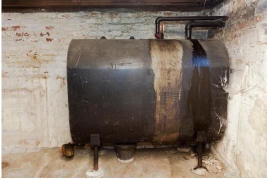
a. Old tanks being removed
