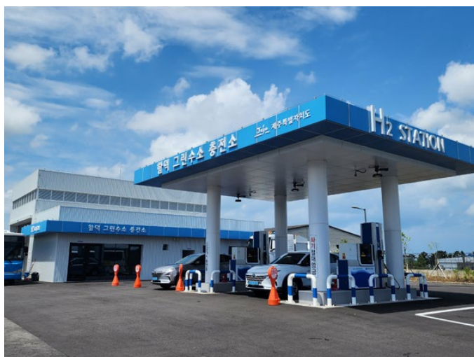
[Hamdeok Green Hydrogen Refueling Station]
