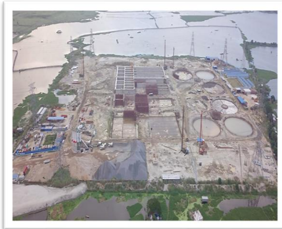
Dasherbandi STP under construction(2019)
