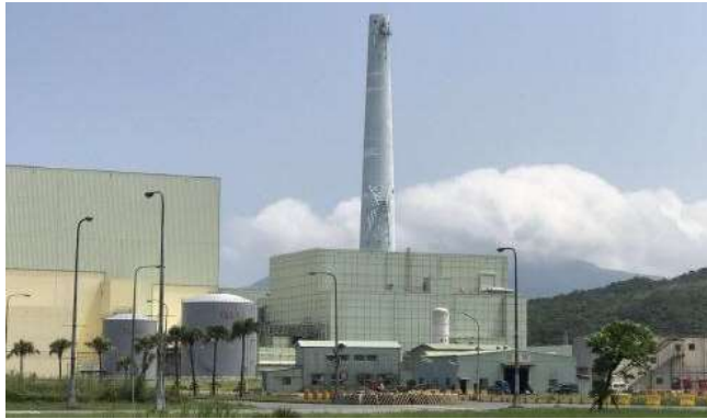
Construction on halt due to opposition
