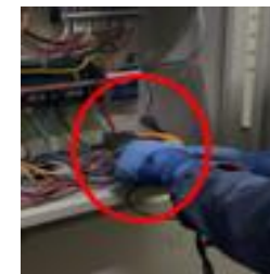
① Connect low-voltage clamp
