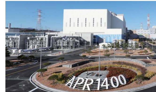
Doosan Enerbility & Saewul Nuclear Power Plant
