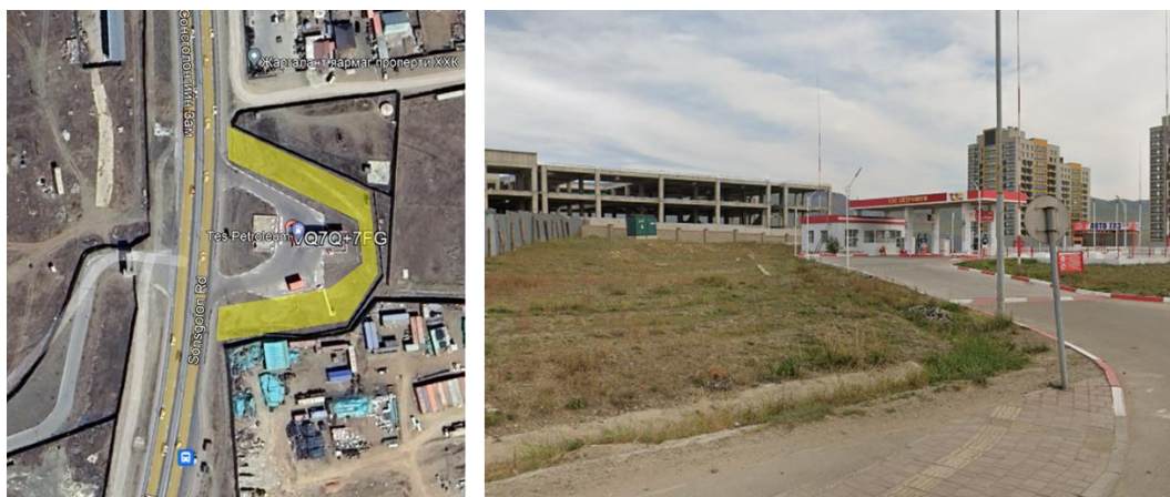
Figure 7-8: Petrol Station TES microgrid fast charging site
