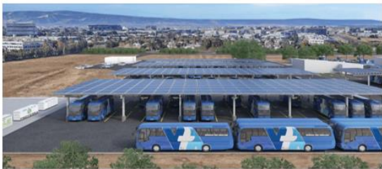
Various suppliers (Siemens, Schneider Electric) offers an e-bus micro grid solution for charging depots. This includes RES.
